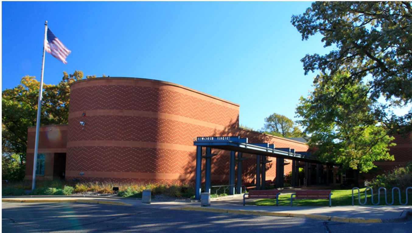
Image 1 – Existing Wentworth Library exterior, main entry walkway
