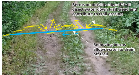
Example of trail in need of debemming at Lebanon Hills Regional Park the trail tread. The increased water volume and velocity will erode the trail.
