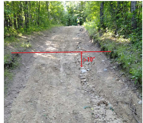
Severe Trail Erosion
