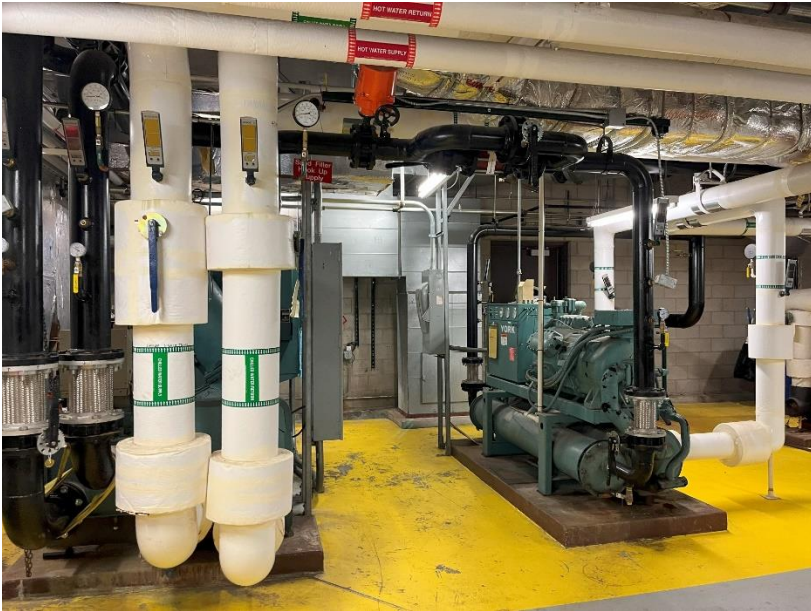
Chillers to be replaced
