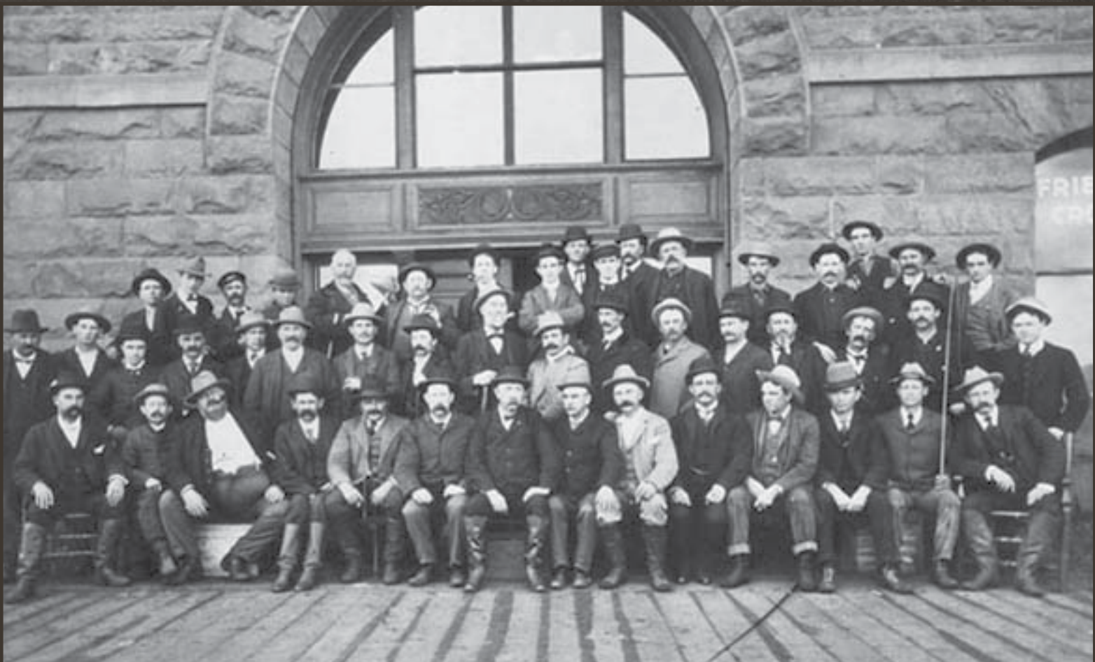
Early workers at the Stockyard Exchange Building, 1898.
